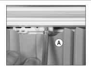
Move the stationary rails flush with their respective end plates. **Note:** To move the stationary rail bracket, pull the bottom of the stationary rail into the room slightly before sliding the bracket. Attach the stationary rail bottom brackets. The brackets may be attached to the sill or floor, or to the jamb using the inside mount adapter.
